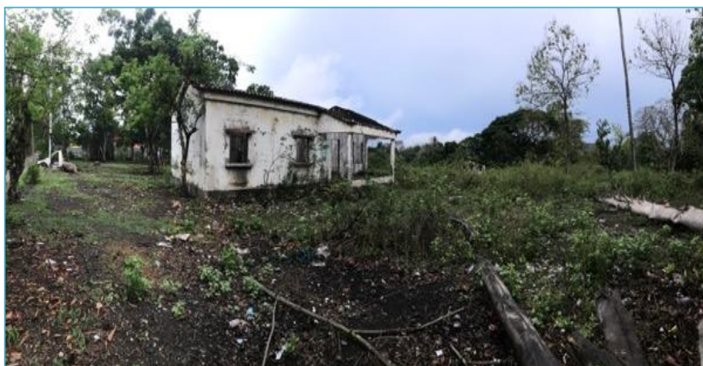
Plate 19- Location of the Letefoho North Tank, abandoned government building that requires demolition prior to construction of the tank.
