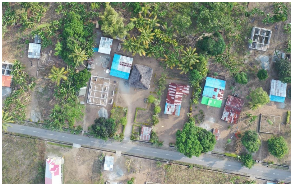
Plate 23 Location of the proposed location of a Public Toilet in Suco Holarua Center
