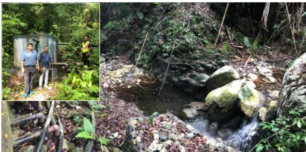
Plate 2- Merbuti River and the existing Intake structure, BPT and pipelines
