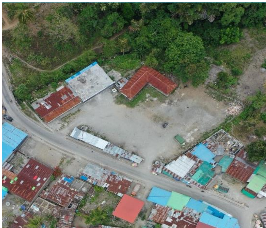
Plate 21- Location of the proposed Public Toilet in a market place in Suco Letefoho
