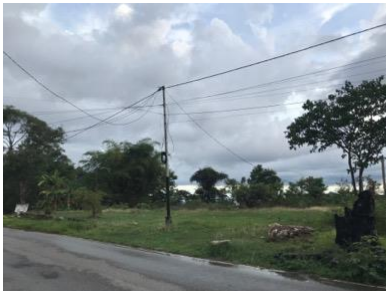
Plate 16- Posto Tower Tank within government compound
