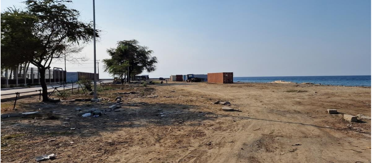
Figure 6-4: Ocean Outfall site, November 2023 (photo credit: B. Lammers)
