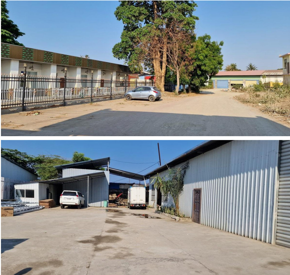
Figure 6-3: WWTP site, November 2023 (photo credit: B. Lammers)
