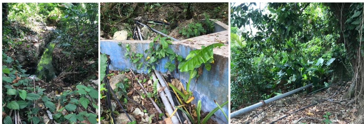
Plate 1- Showing Loihuno Spring, the intake box and existing transmission pipes
