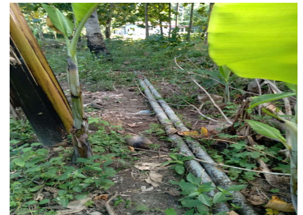
North view of transmission mains to be rehabilitated (Sub zone 3.4)
