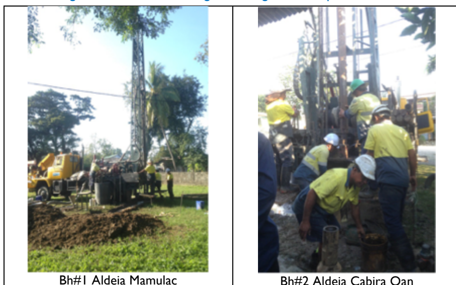
Figure 7 - Borehole Testing in 4 Designated Prospection Points
