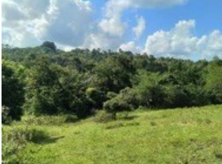
South view of the Proposed Area. Unstable slope
