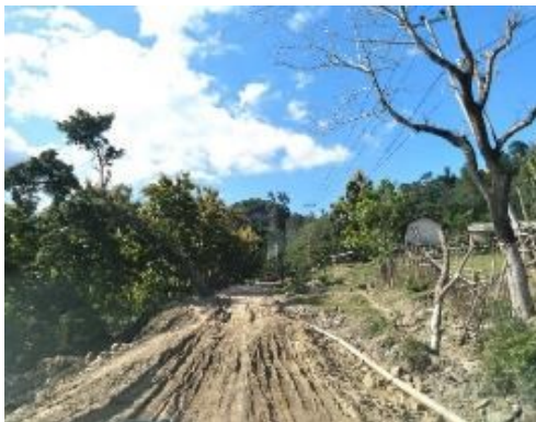
Northward is the existing transmission main (pipeline on the right side) from main source Loihuno I spring to be rehabilitated, Suco Loihuno (outside distribution zone)
